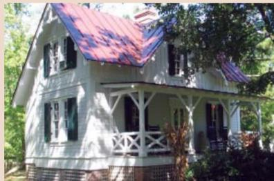
A new standing-seam metal roof was recently completed on the little keeper's house. The new roof replicates the house's original roof.
